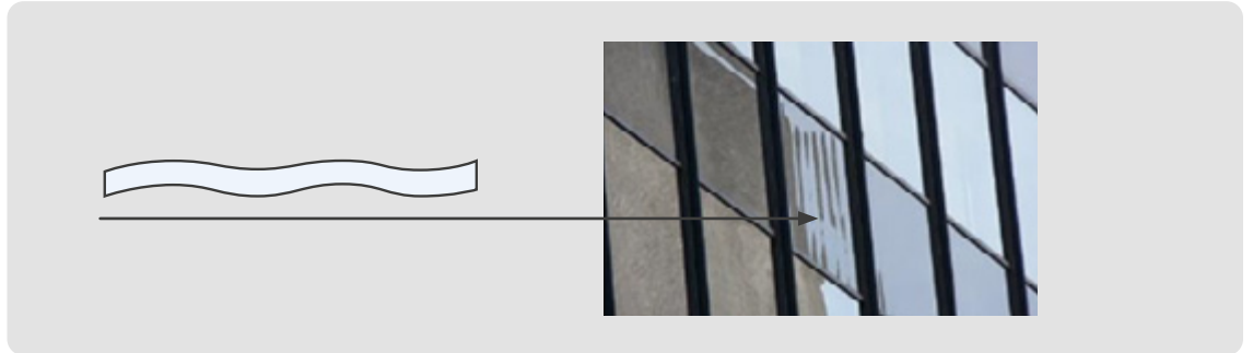
d) Measurement of concavity and convexity of the insulating glass unit according to EN1279: G5 Specification: no limit, natural phenomenon.
