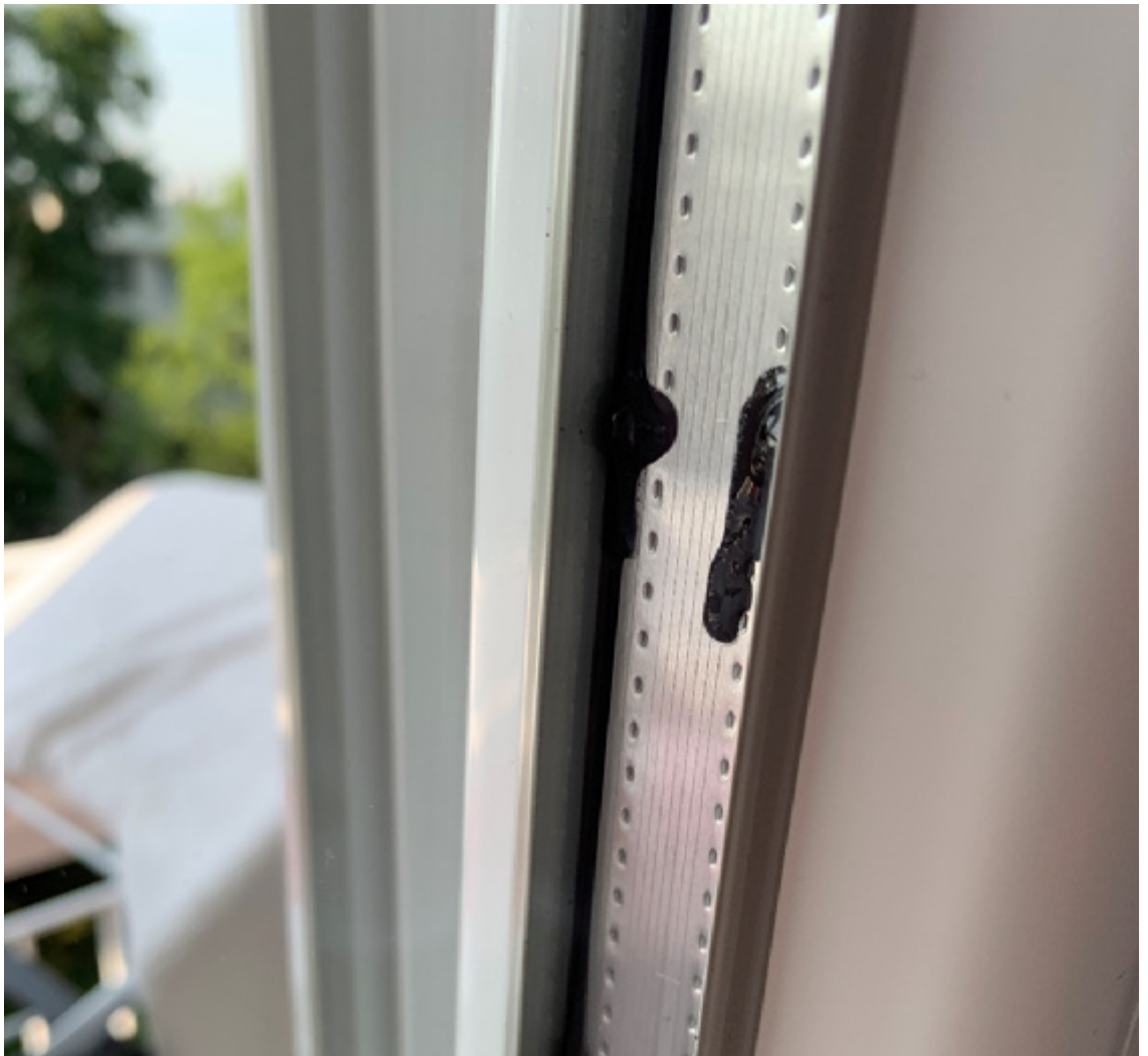
Fig 21 The effect of using incompatible materials.
